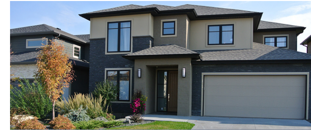
Zero-step entrance into the home
